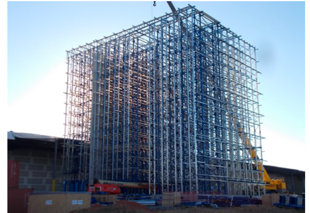
HOCHREGALLAGER IN SILOBAUWEISE AUTOMATED CLAD-RACK WAREHOUSE
